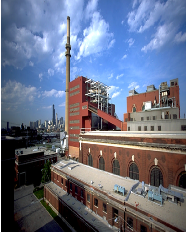
Fisk Generating Station
